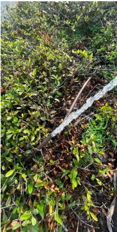
Cut drip tube in plant bed east of 301 entrance
