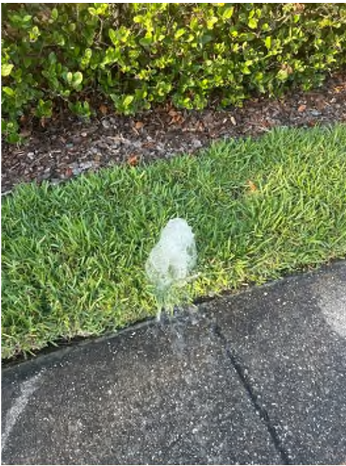
Zone A16 – Replaced broken sprinkler
