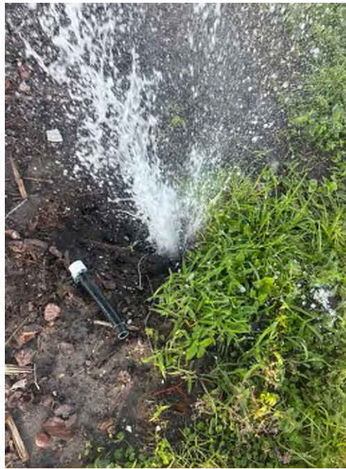
Zone A17 – Repaired cut in funny pipe
