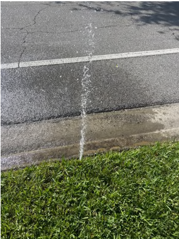
Zone B35 – Replaced broken rotor
