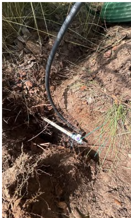
Installation of new tree bubbler at Hadden Mist
