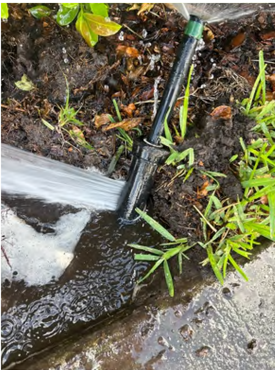
Zone A26 – Replaced cracked sprinkler
