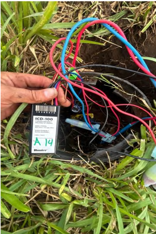
Zone A14 – New decoder and solenoid
