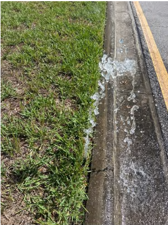
Zone B45 – Replaced broken pop-up
